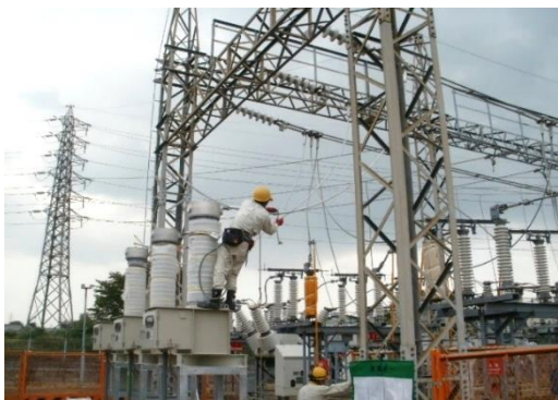
計器用変圧器取替
