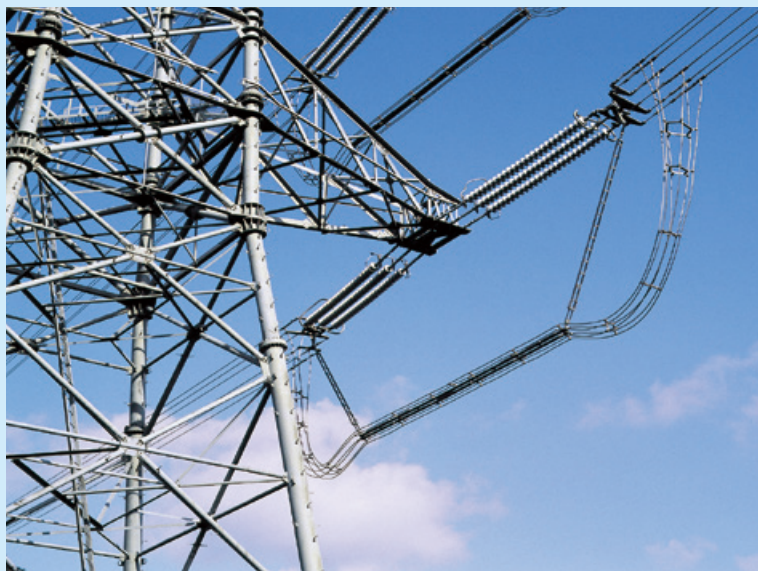
▲ 6導体用吊架式ジャンパ装置 Hang-up Jumper device for 6-bundle conductor
