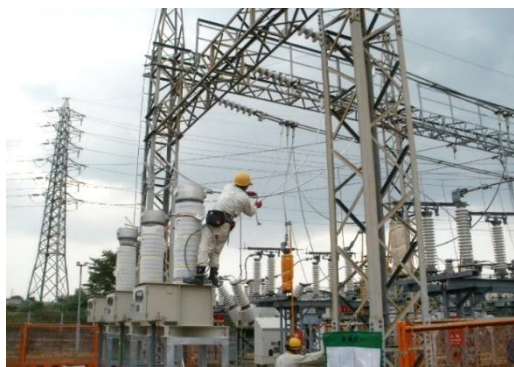
計器用変圧器取替
